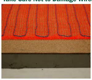
5. (B) Attach Free Form Type Wire Systems Using Manufacturers Recommended Fasteners. Take Care Not to Damage Wires.
