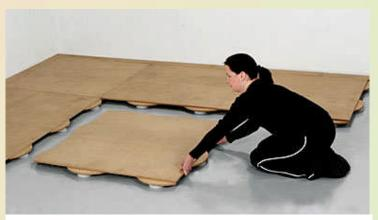
The 42" x 42" Rosco SubFloor panels lock into each other seamlessly. Perimeter pieces lock the entire floor together.
